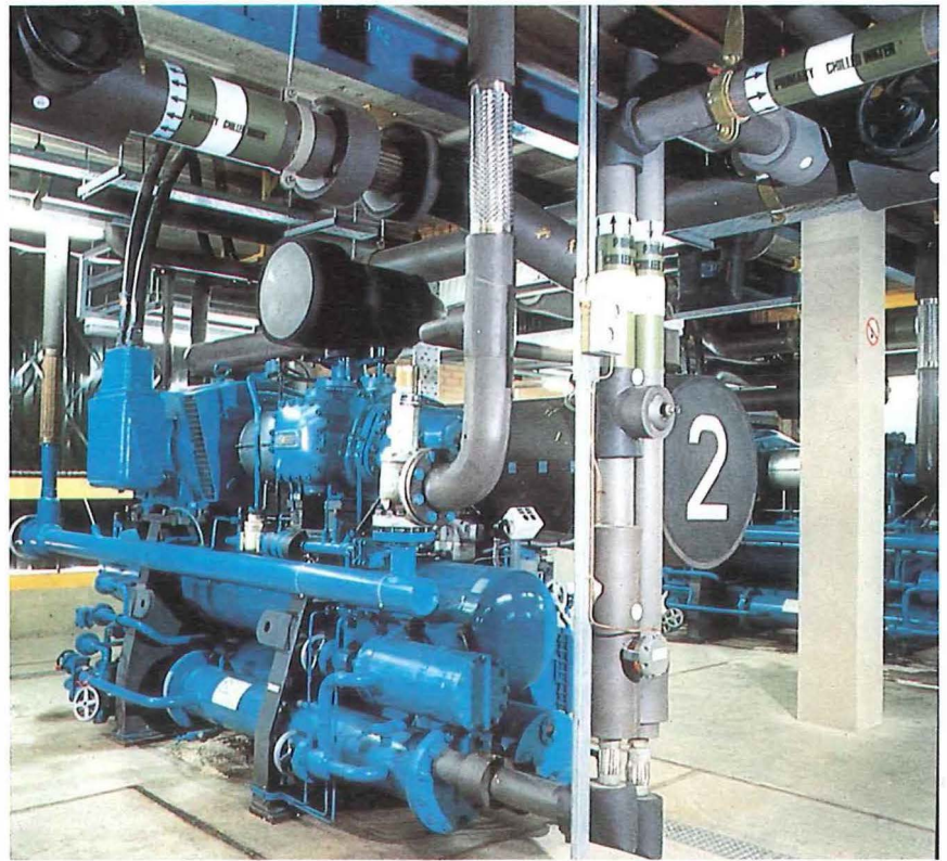
Figure 1—Example of central chilling plant
