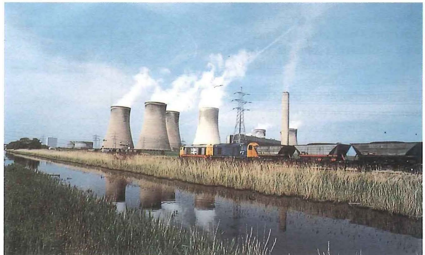
Figure 1—A typical electricity generating station (Photograph courtesy of the Electricity Association)
