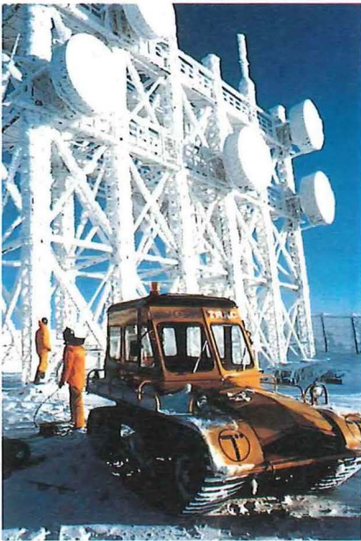
Figure 11—Power plant must work in all conditions
