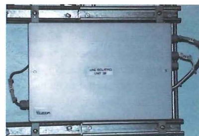
Figure 7—Line Isolating Unit 3B
