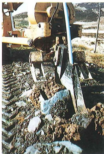
Figure 2—Vibrating head working in rocky location
