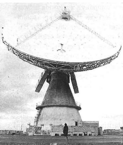
Goonhilly satellite earth station
