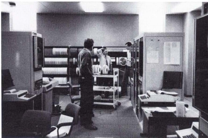
Figure 1—Routing and billing centre (RBC) computers in a CMC exchange. Note the 'computer room' environment
