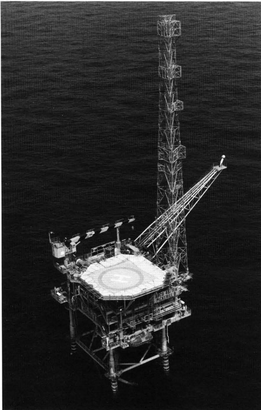
Figure 6—Pickerill B platform
