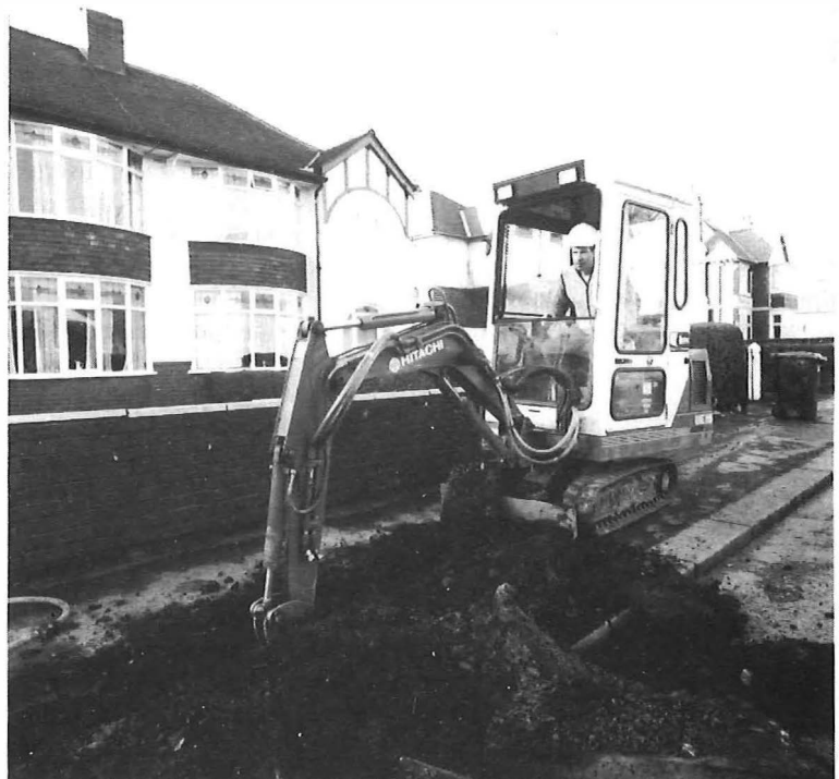
Excavating a trench using a mini-excavator
