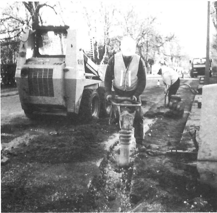
Compacting a back-filled trench
