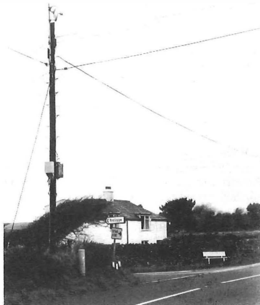
Figure 3—Camelford multipoint system—pole-mounted outstation
