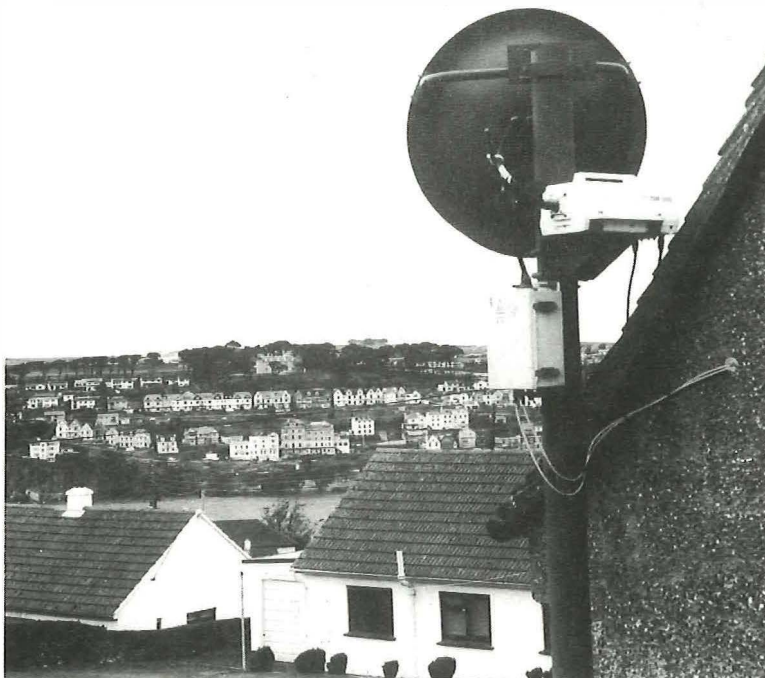
Figure 1 19 GHz radio at Polruan remote concentrator unit
