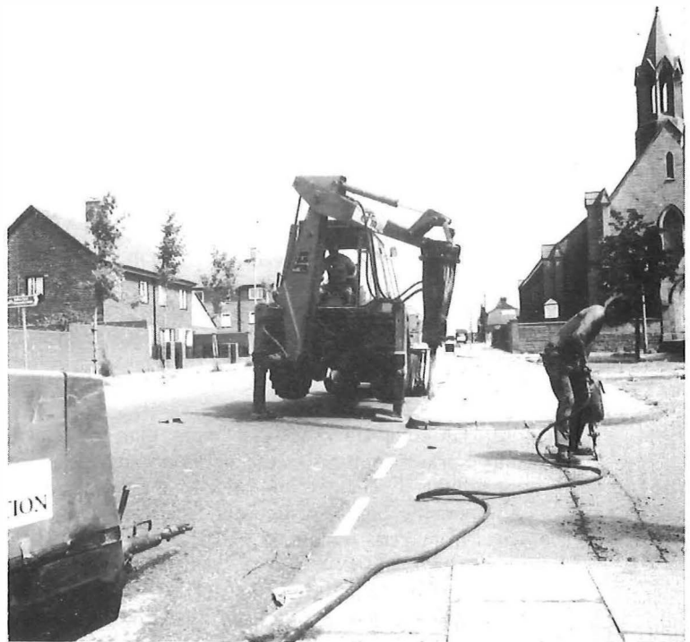
Cutting a road crossing
