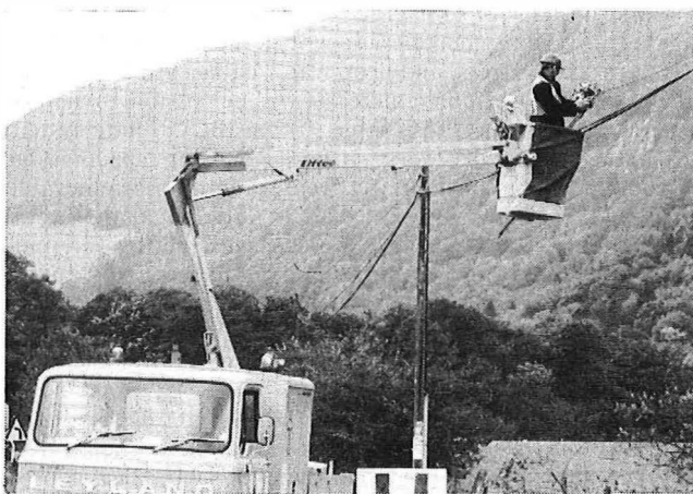
FIG. 14—Installation of overhead optical-fibre cable in Wales
