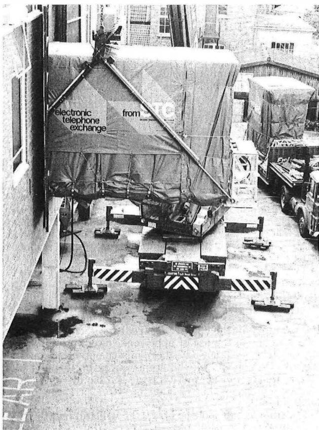
FIG. 1—A module being manoeuvred into the apparatus room
