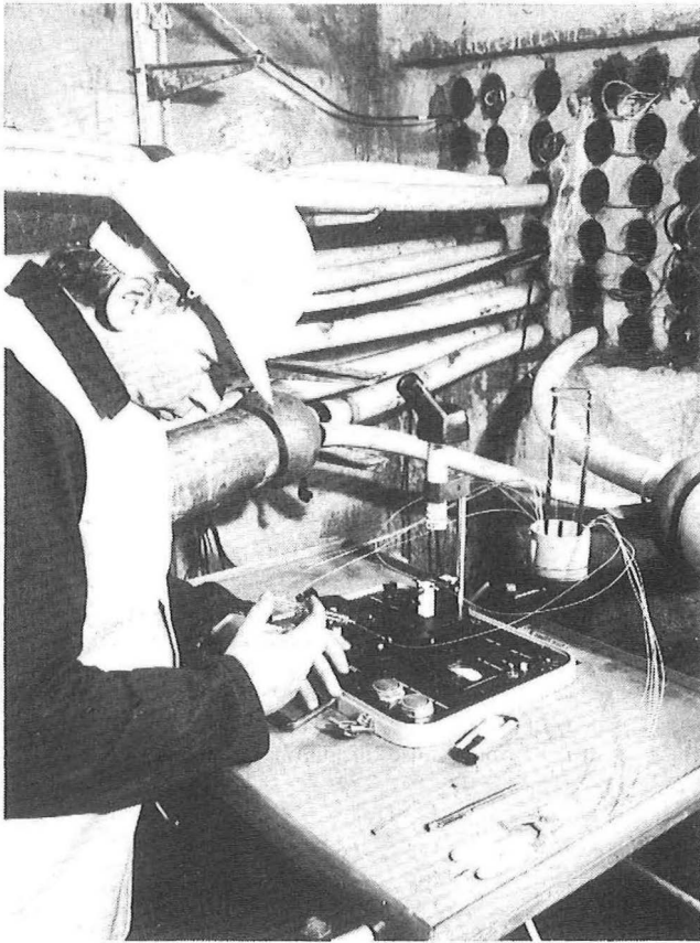
FIG. 9—Fusion splicing on one of the proprietary 8 Mbit/s routes in London
