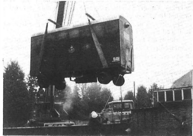
Mobile telephone exchange being lifted over the stone wall
