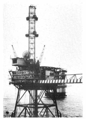
FIG. 1-Typical steel-type production platform
