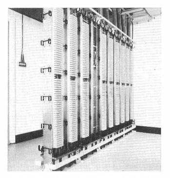
FIG. 8—Frame Distribution No. 105A used as a double-sided TJF for a large digital PABX
