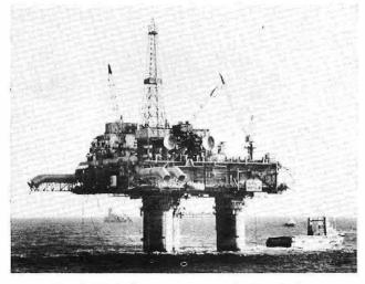
FIG. 2-Typical concrete-type production platform
