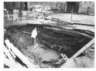
FIG. 1-Initial support given to the duct line
