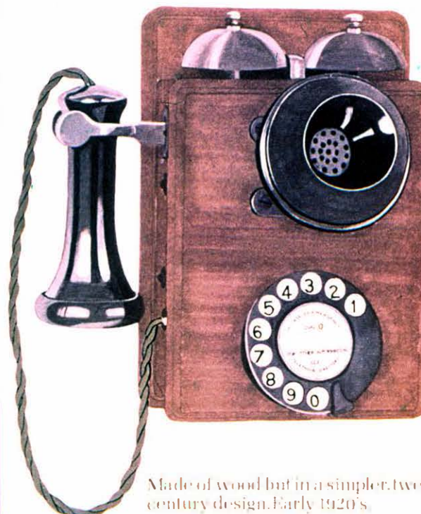
Handsets gave freedom of movement to telephone users, but early handsets needed individual batteries and were not successful when electricity was fed from the exchange, 1900.
