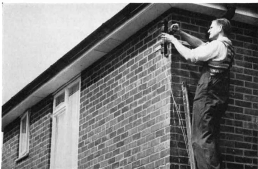
Fixing telephone wires to a customer's house
