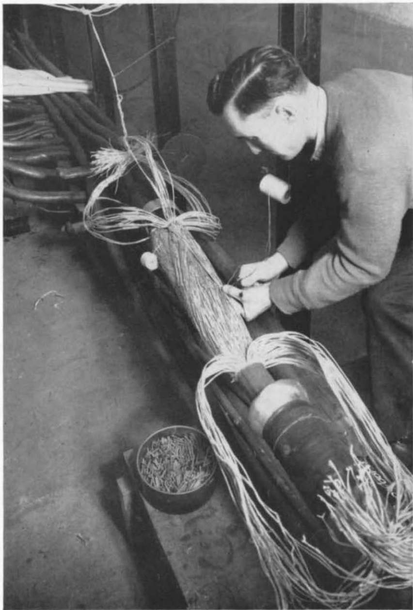
Joining up a big cable
