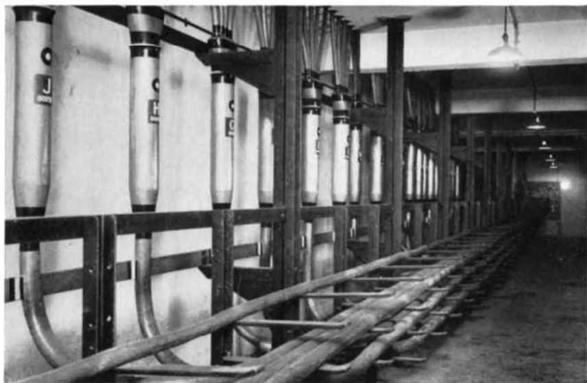
Cables coming into a big telephone exchange
