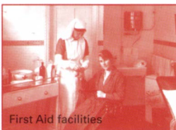
First Aid facilities
