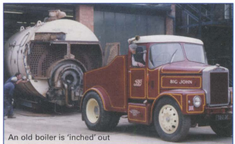
An old boiler is 'inched' out
