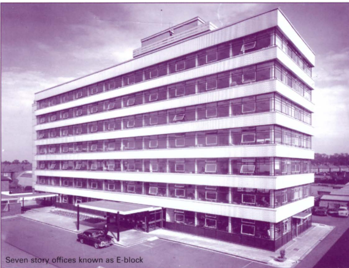
Seven story offices known as E-block
