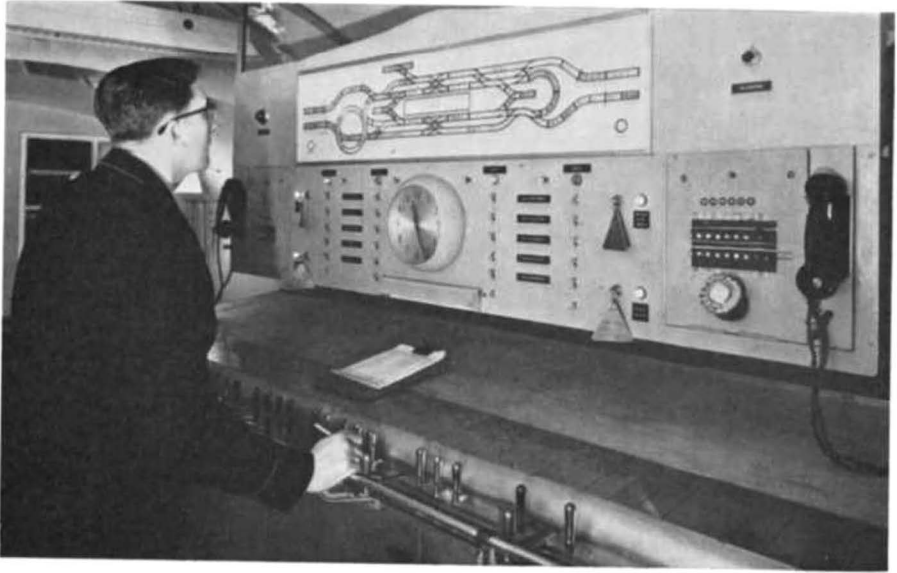
Post Office Railway: control cabin
