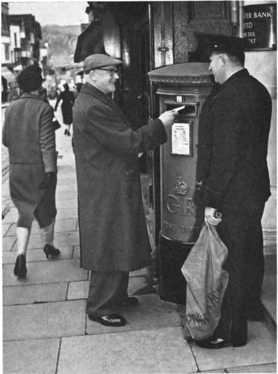
Catching the post: the box about to be cleared
