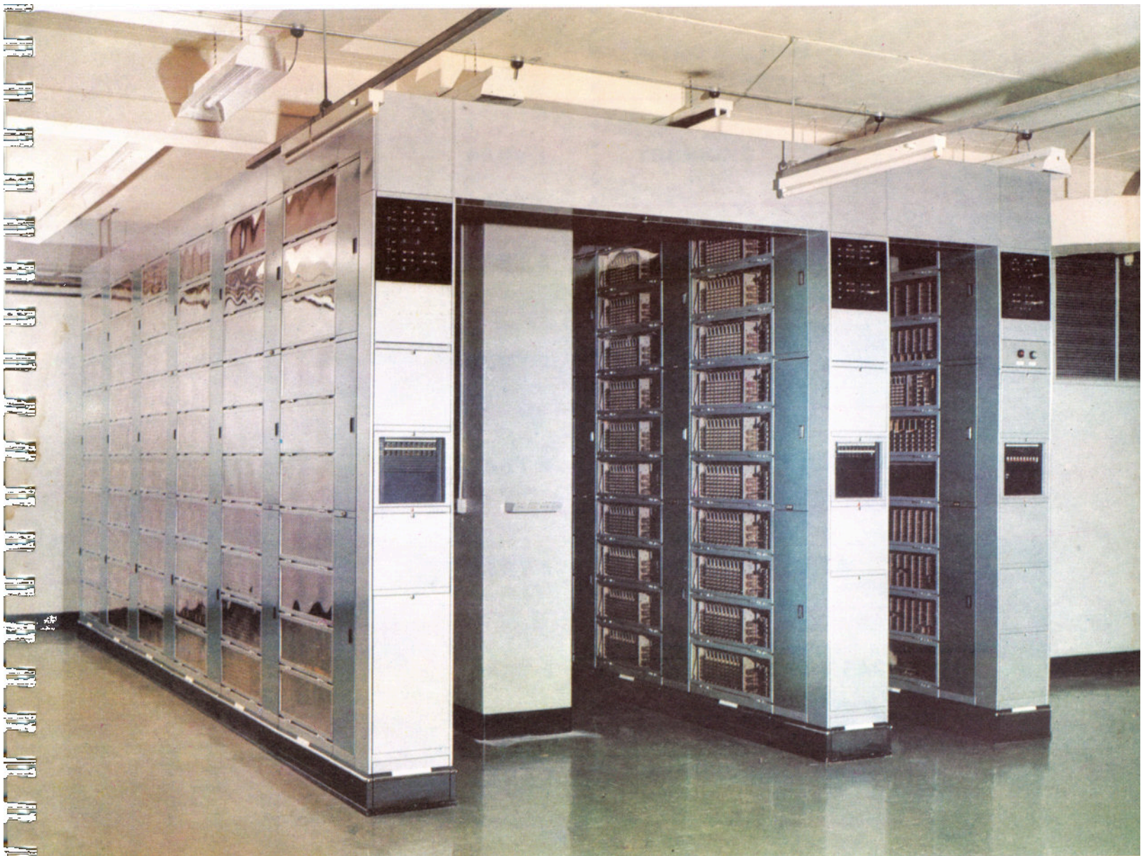
GATEWAY EXCHANGE, SYDNEY, AUSTRALIA. —This exchange is the 4-wire switching centre terminating the Commonwealth Pacific cable. It permits operators in all the main switching centres in Australia to dial direct to subscribers in North America and Great Britain, using high-speed v.f. signals. It also provides for operators in Great Britain and North America to dial direct to subscribers throughout Australia.
